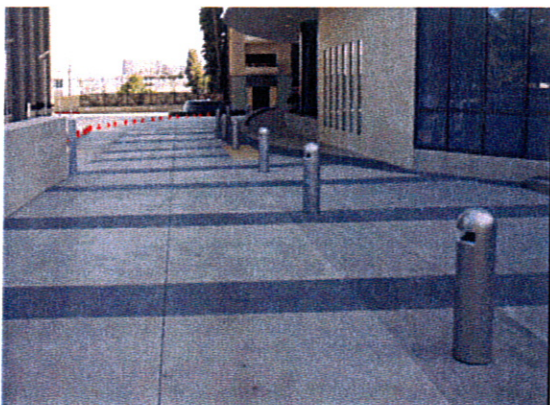
Various lighting methods including bollard lighting for pedestrian sidewalks
