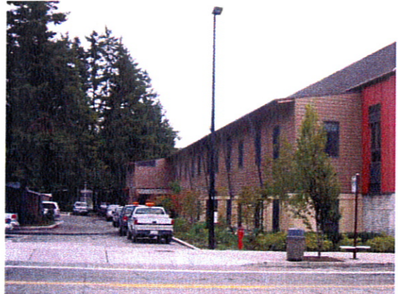
Parking to the side of the building
