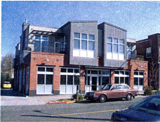
Rely on building massing and materials to place a strong visual emphasis on the street; upper level is both set back and broken up into separate volumes to reduce the perceived scale of the building
