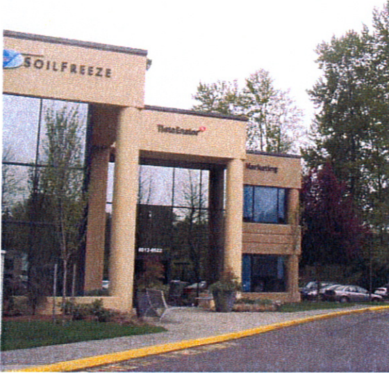
Double height glazing, columns and landscaping give prominence and identity to a main building entrance
