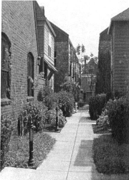
Connections provide safety and comfort through large sites
