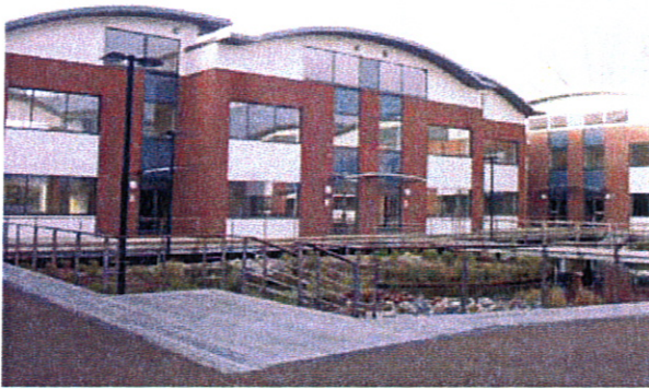
Example of simple modulation with deep openings that create shadow lines, provide visual relief that is carried to the top of the building.
